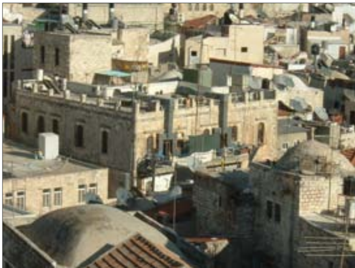
Fig. 5-24: The incompatible add elements by the settlers to the original facades in the Old City of Jerusalem. (researcher).
