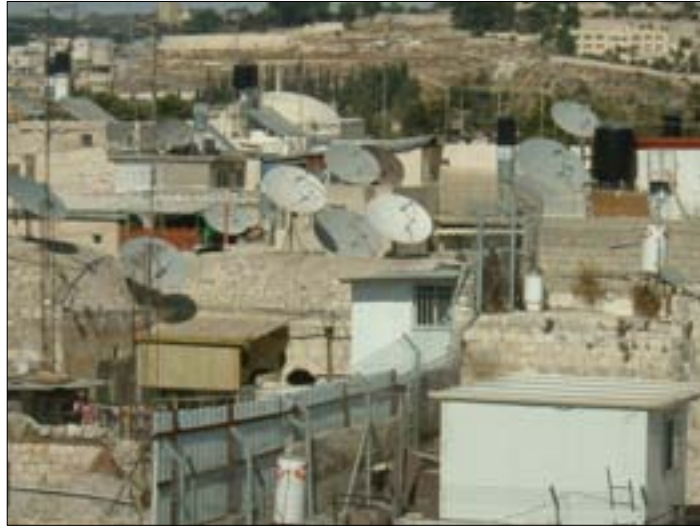
Fig. 5-21: The added modern services which influence the total city form in Jerusalem Old City (researcher).
