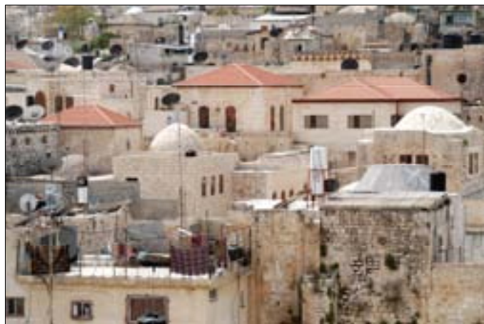
Fig. 5-22: Using different roofing systems between pitched, domed, & flat roofs in Jerusalem Old City (researcher).
