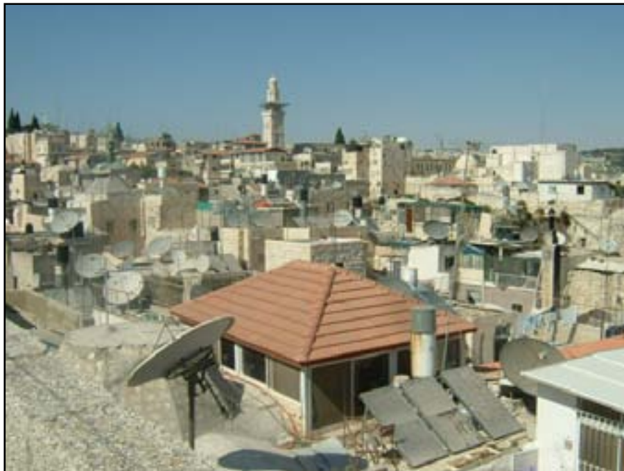
Fig. 5-15: Covering the open courtyards with new masses and covering systems in Jerusalem Old City (researcher).
