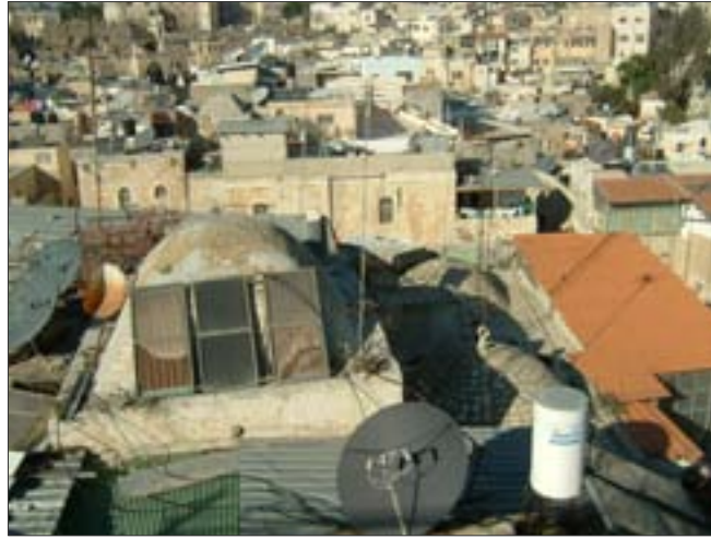
Fig. 5-23: Using different roofing materials which influence the whole city image in Jerusalem Old City (researcher).
