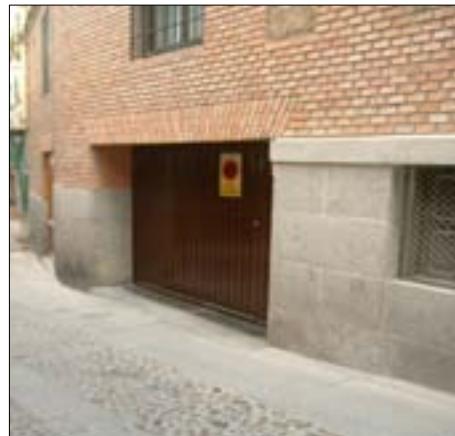
Fig. 6-12: Parking inside the houses in Toledo Old City (researcher).
