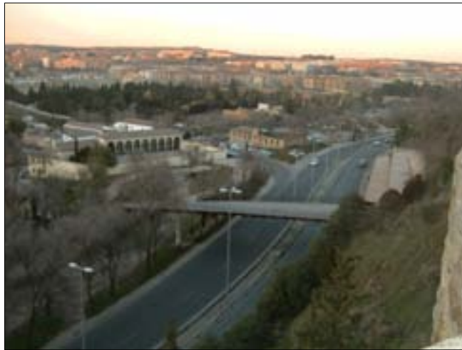
Fig. 6-14: Connecting some public services from outside the Old City of Toledo by modern axis (researcher).
