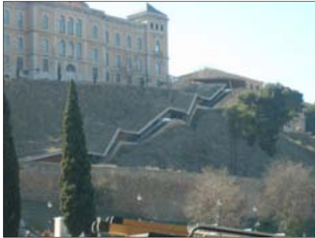
Fig. 6-13: Using high- tech (electrical stairs) means in order to offer pedestrian axis from outside tourist parking to inside the Old City of Toledo (researcher).
